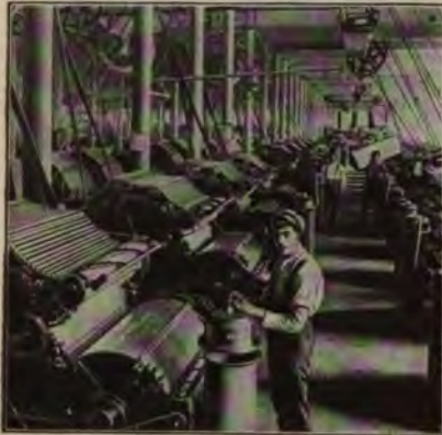
Photographs of a cotton mill in Columbia, S. C., showing four steps in the manufacture of cotton goods. 1. The carding machine straightens the fiber and rolls the cotton, which is gathered into cans.
